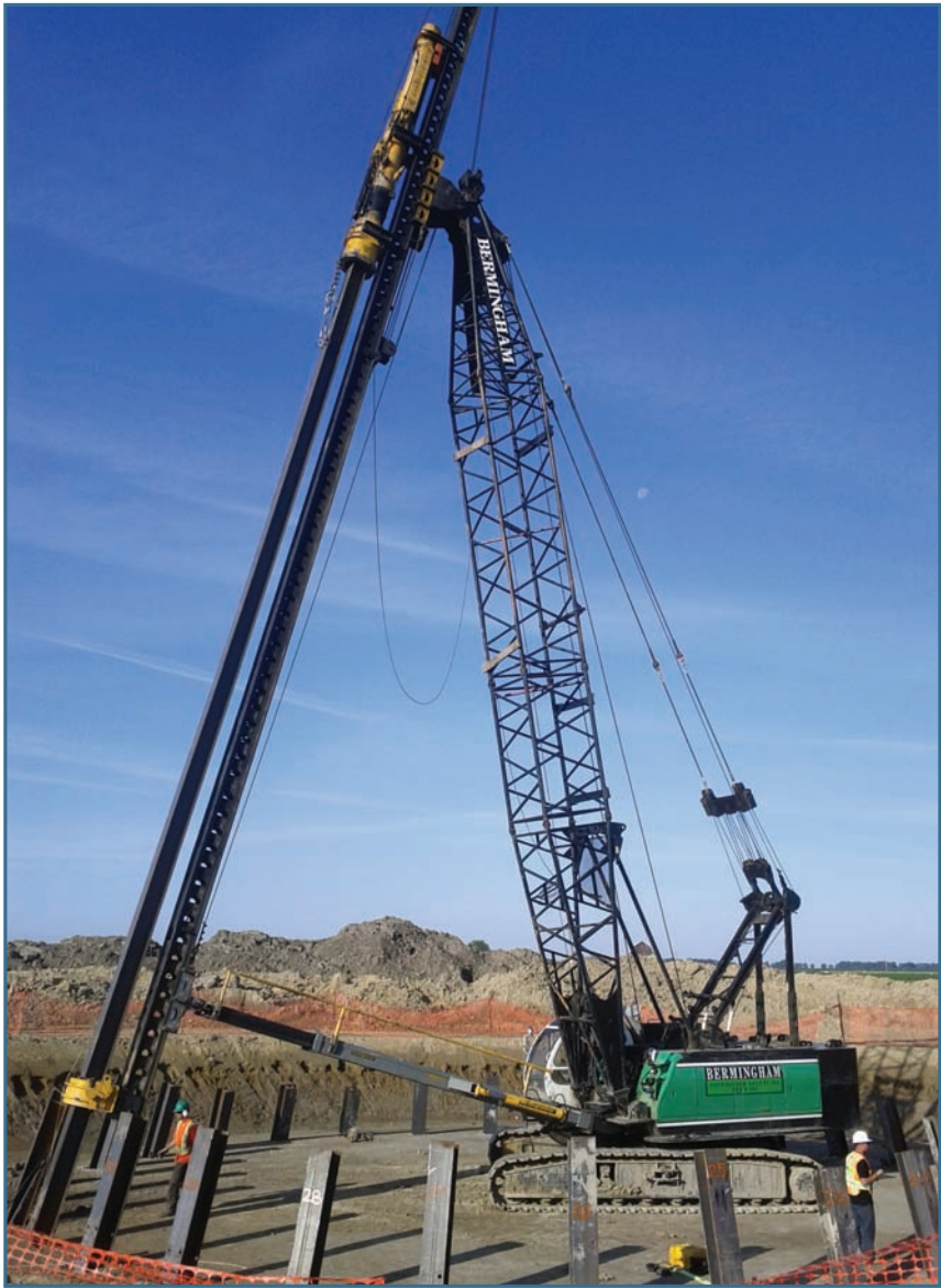
▲ Vertical Travel Leads with B32 Diesel Hammer on 1:4 fore batter alignment
